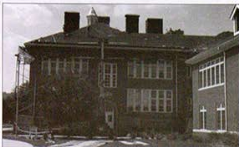
Crews work on the roof of Mount Kisco Elementary School during the waning days of summer to get the building ready for last week's opening.
